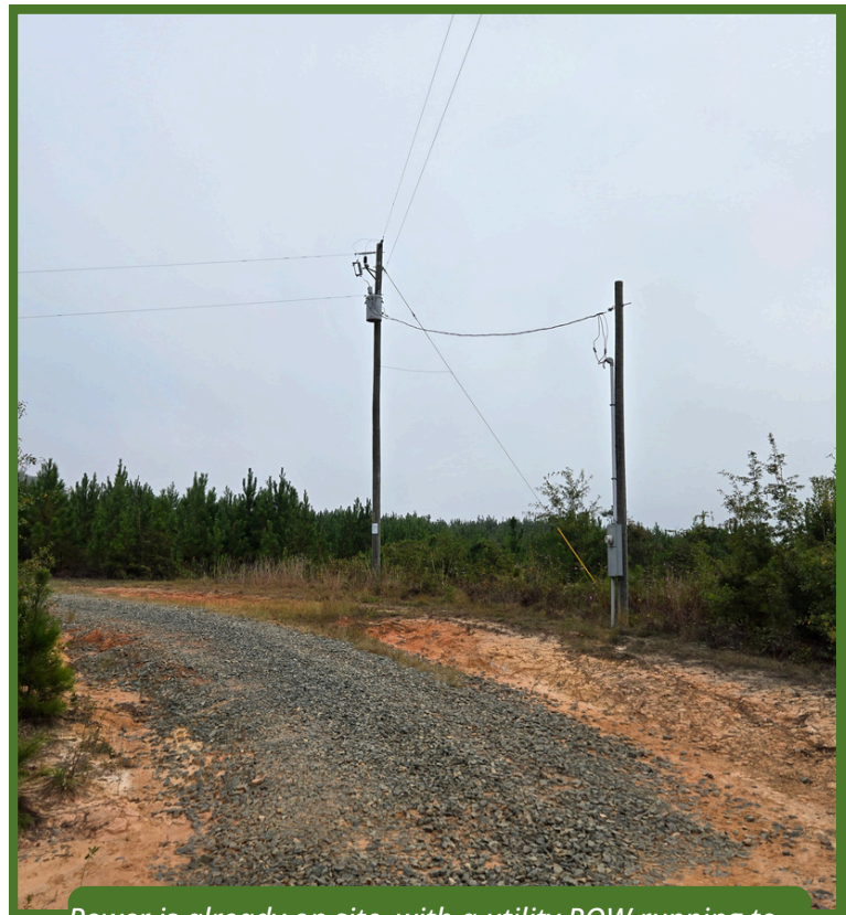
Power is already on site, with a utility ROW running to and through the southwest corner of the tract.
