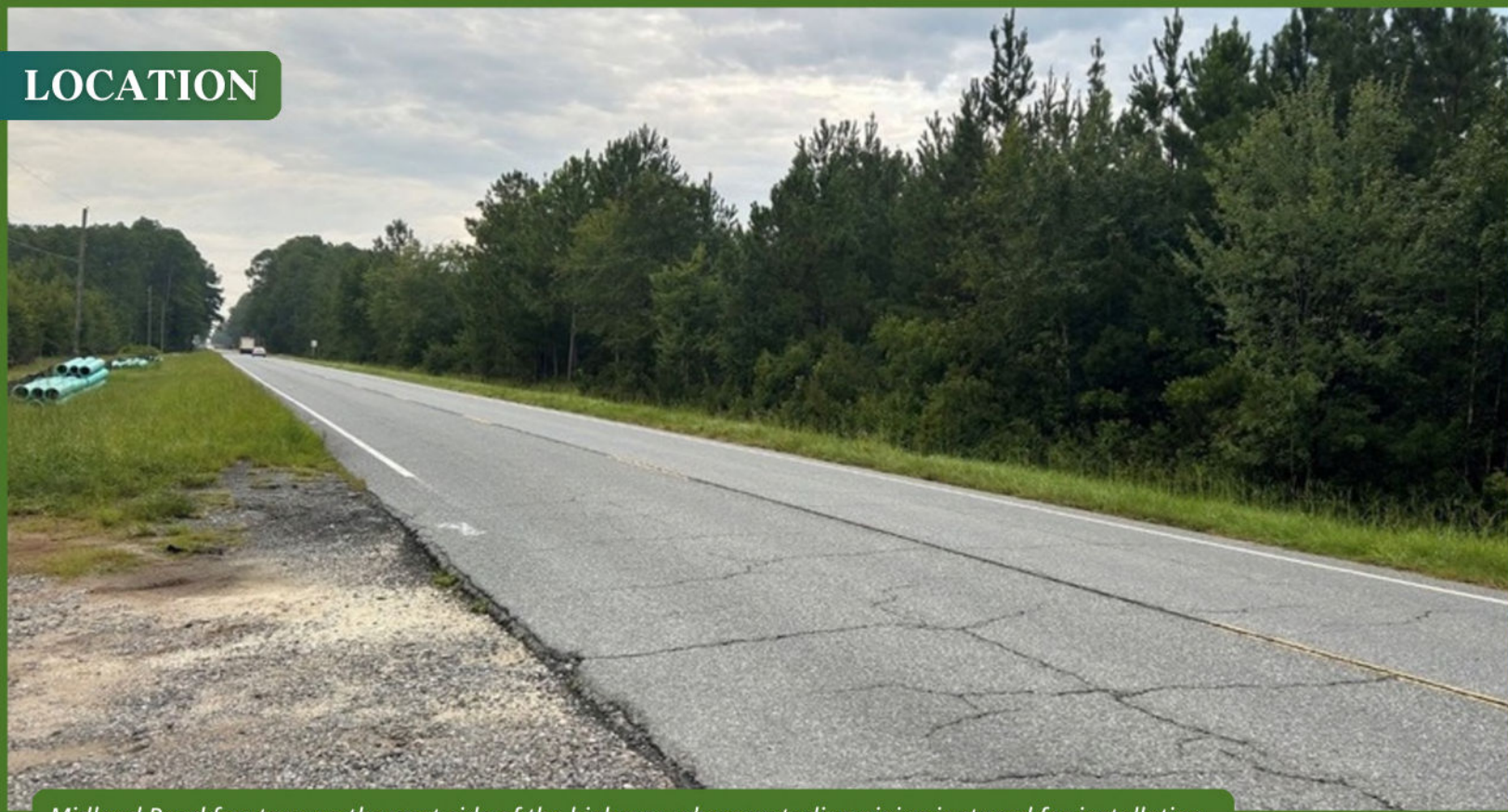
Midland Road frontage on the west side of the highway, where waterline piping is staged for installation.
