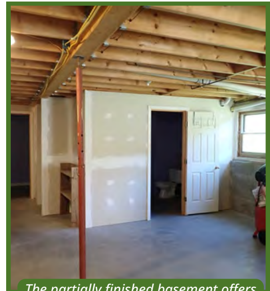
The partially finished basement offers room for additional living space or equipment storage.
