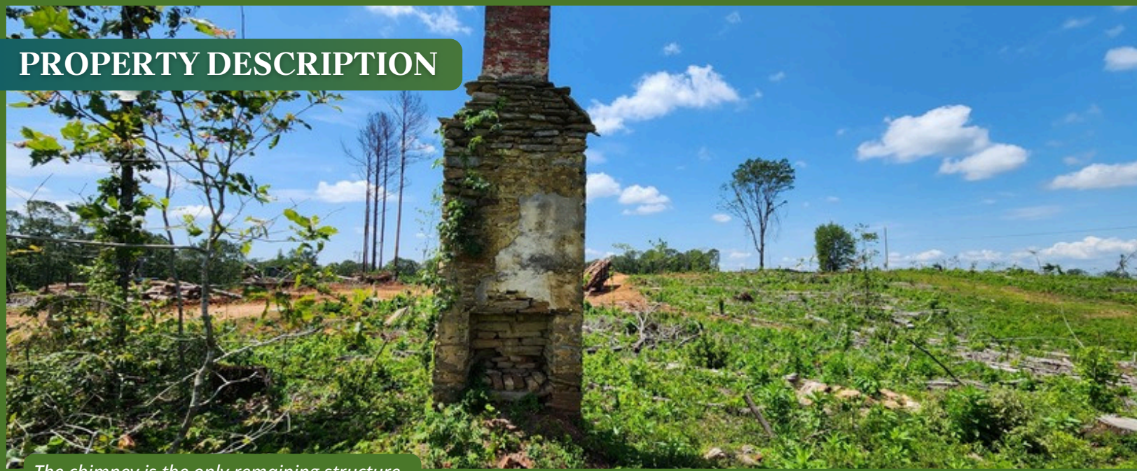
The chimney is the only remaining structure.
