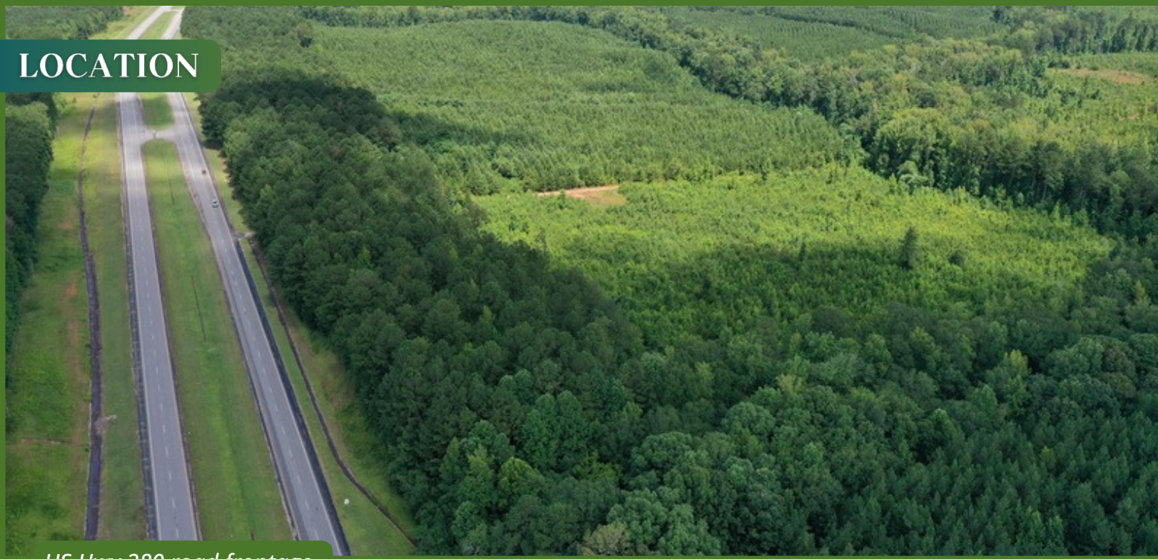
US Hwy 280 road frontage.
