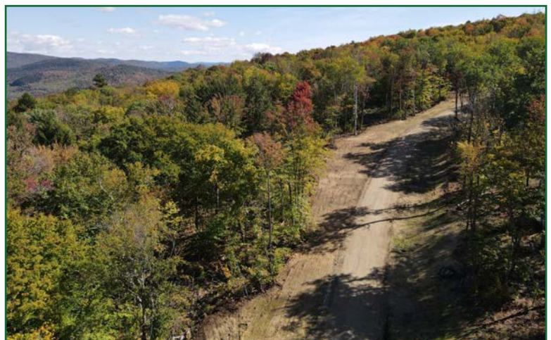
The 20 foot wide access road near the bottom of the subdivision with Lot 2 on the left and Lot 5 on the right.
