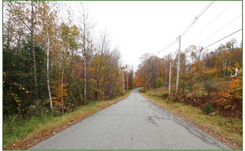
Mine Road frontage with electric poles and the property on the left.
